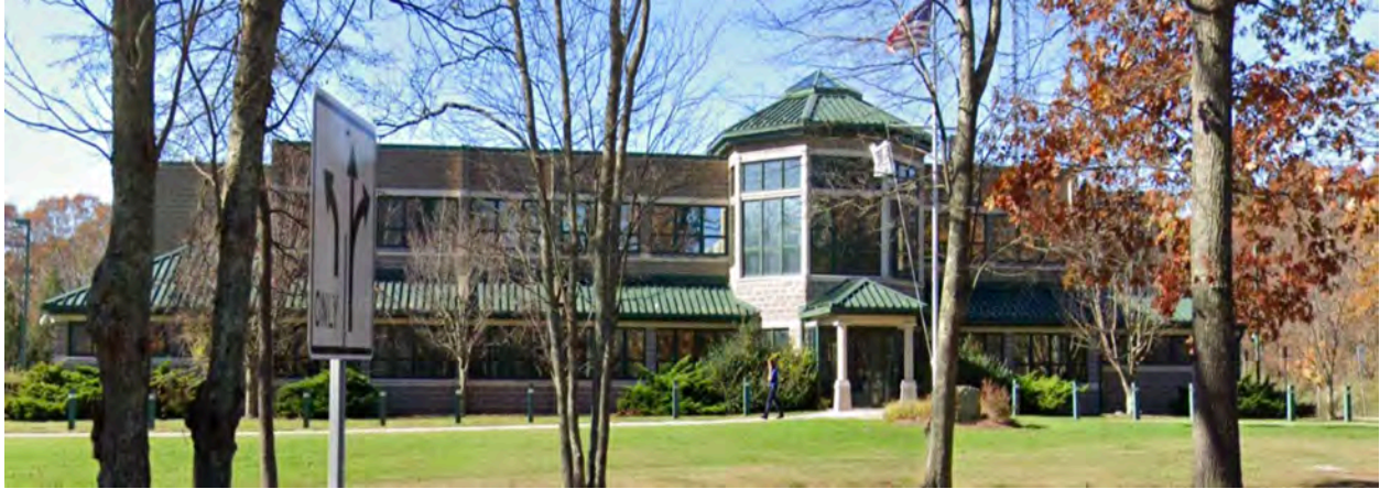
[Public Safety Complex (Credit: Google Earth)]
