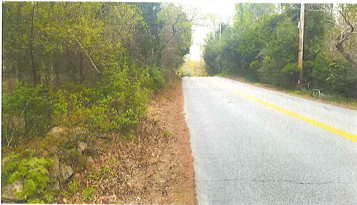
Existing Bar Way Looking North – Sight Distance Restricted by Road Grades / Vertical Curve
