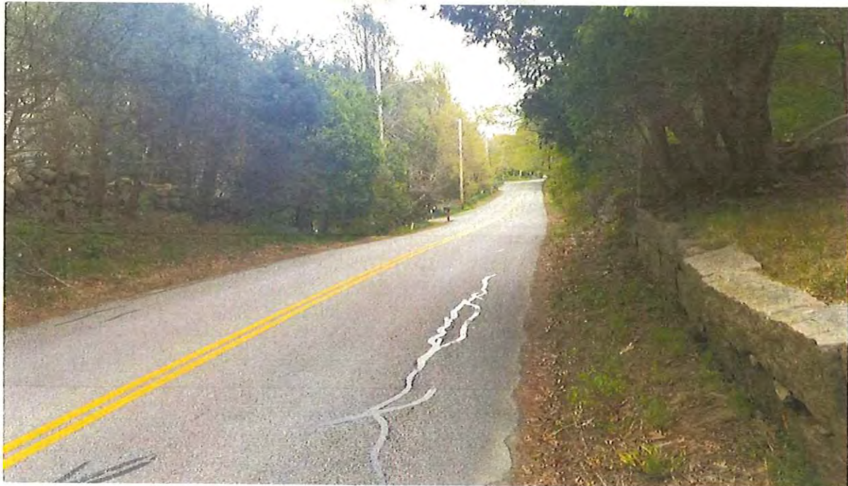
Cemetery=Crest of South Road Vertical Curve (Looking South)
