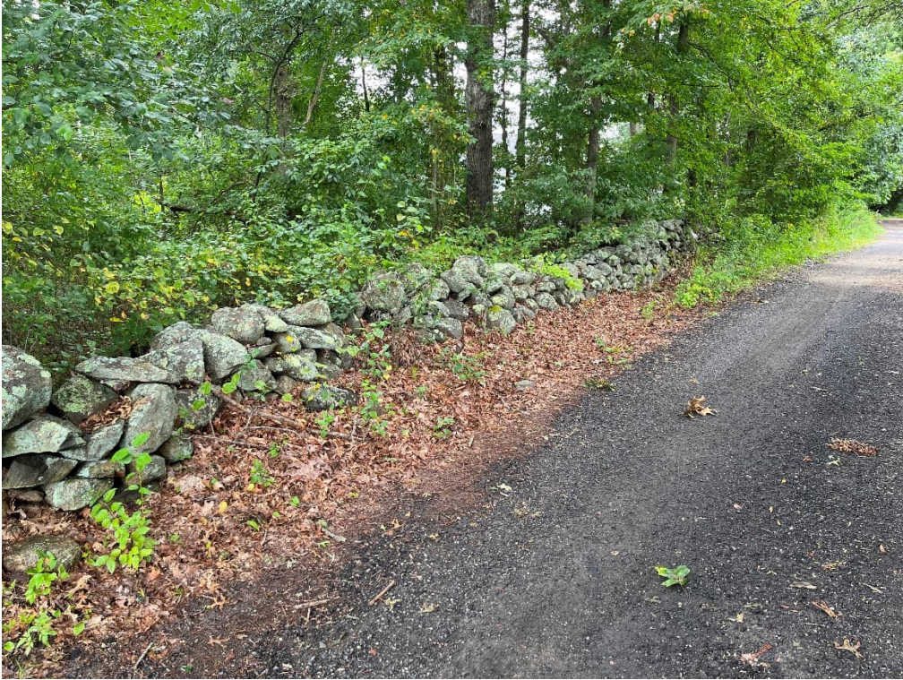
Photo above showing the stone wall and driveway along the southern property line.
