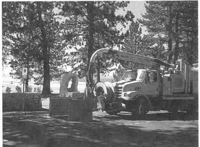
A vacuum truck excavates pollutants from the systems.
